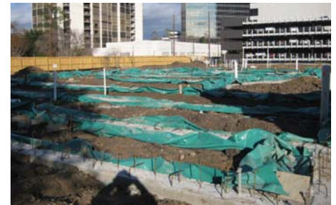
Grade beams have been poured at the new The Youth/Young Adult and Scout Facility (a little muddy after the heavy rain).
