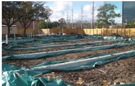
Grade beams have been poured at the new The Youth/Young Adult and Scout Facility (a little muddy after the heavy rain).
