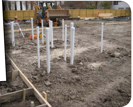
Here one can see the underground plumbing rough-in for the men's and women's restrooms in the new Youth and Young Adult Facility.
