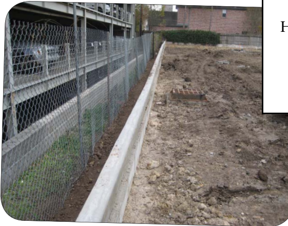
The retaining wall along the east property line has been completed and is ready for backfill.
